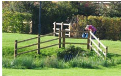
ILLUSTRATIVE EXAMPLE OF TIMBER POST AND RAILS TO BE IMPLEMENTED TO THE TOP OF HEADWALLS TO PREVENT FALL HEIGHT ISSUES
