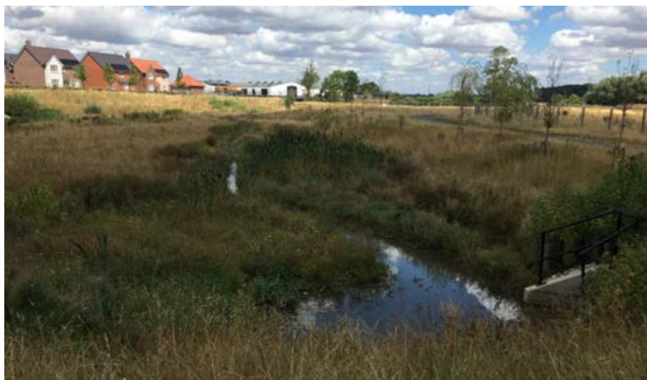
WESTERN EDGE GREEN - SUDS BASIN WITH WATER CHANNEL
