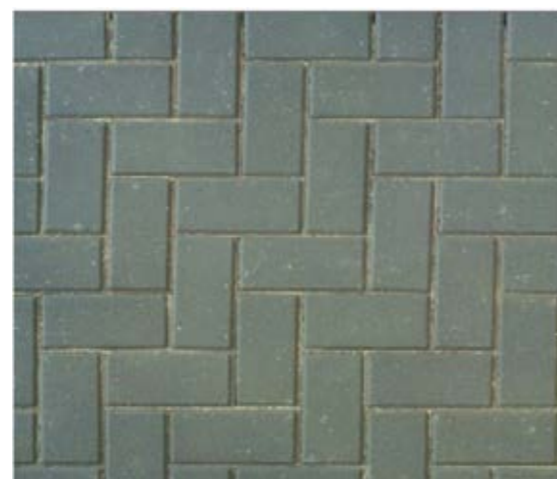
SHARED SURFACES – BLOCK PAVING – COLOUR: GREY
