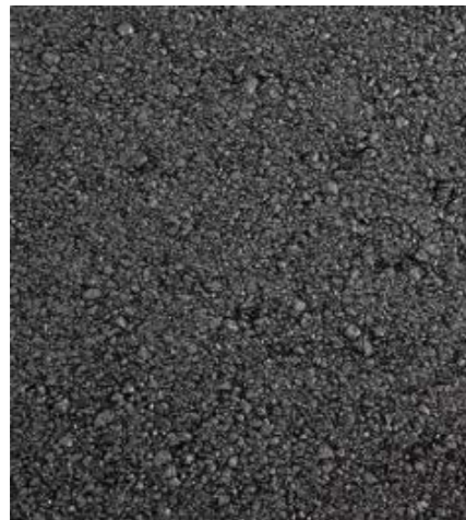
MAJOR ACCESS ROAD – STANDARD TARMAC
