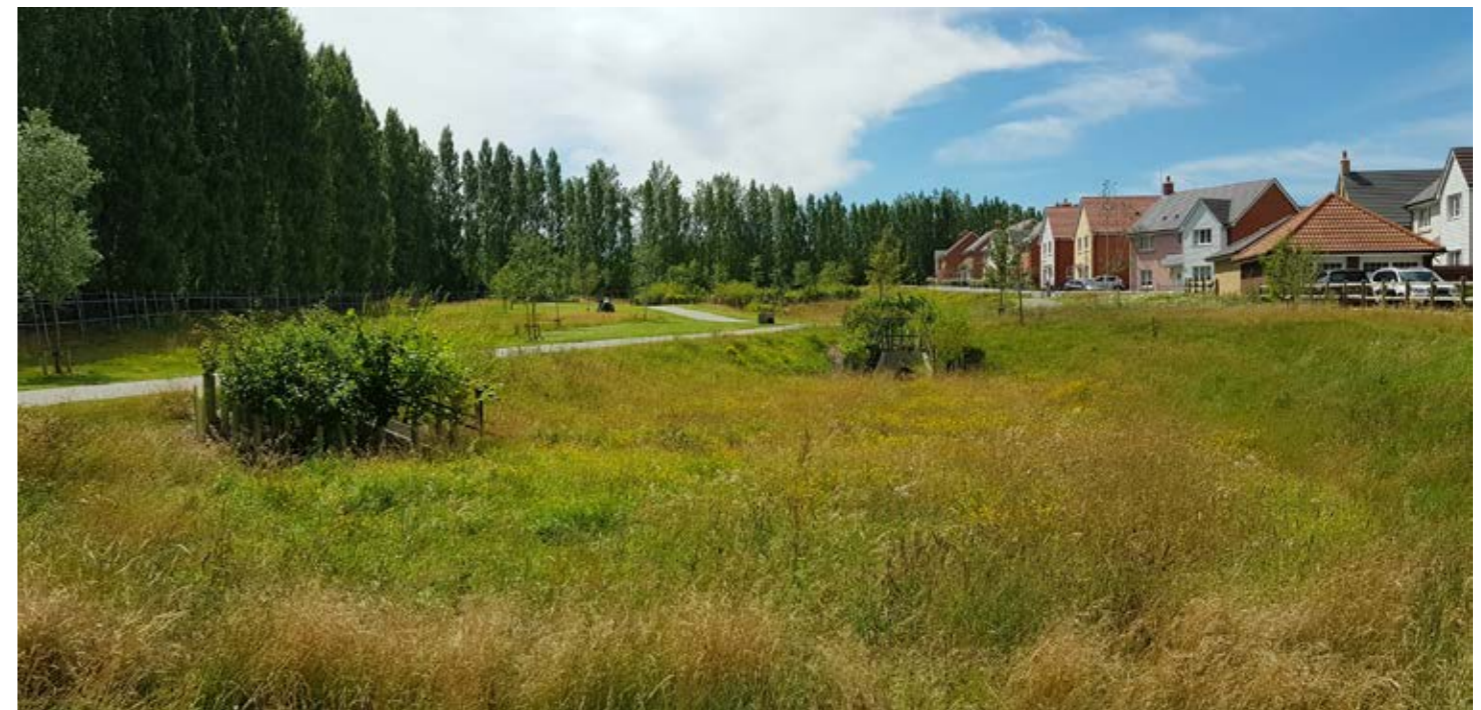
ATTENUATION BASIN (DAVENTRY) – AFTER ESTABLISHMENT OF LANDSCAPE
