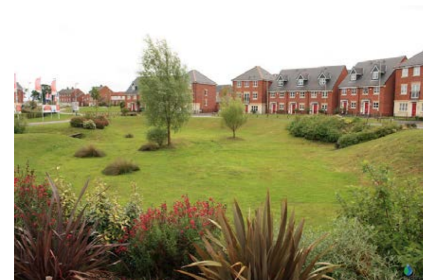
WELL-OVERLOOKED ATTENUATION BASIN
