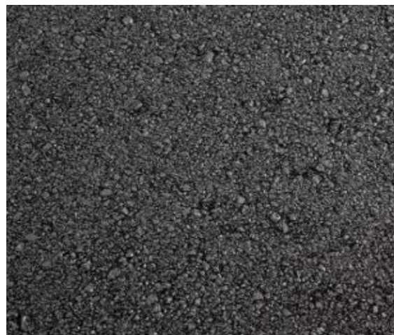
MINOR ACCESS ROAD – STANDARD TARMAC
