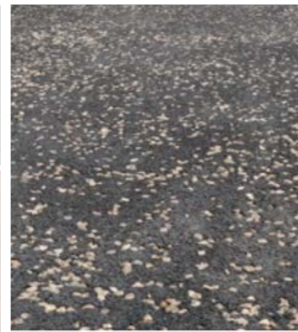
FOOTWAY/CYCLEWAY – HERITAGE FINISH TARMAC (BUFF CHIPPINGS)
